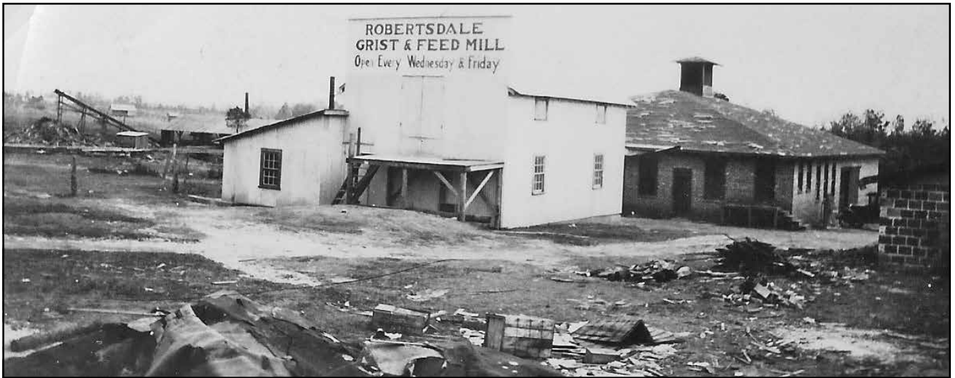
Photos show the expansion of the Robertsdale Grist & Feed Mill.
