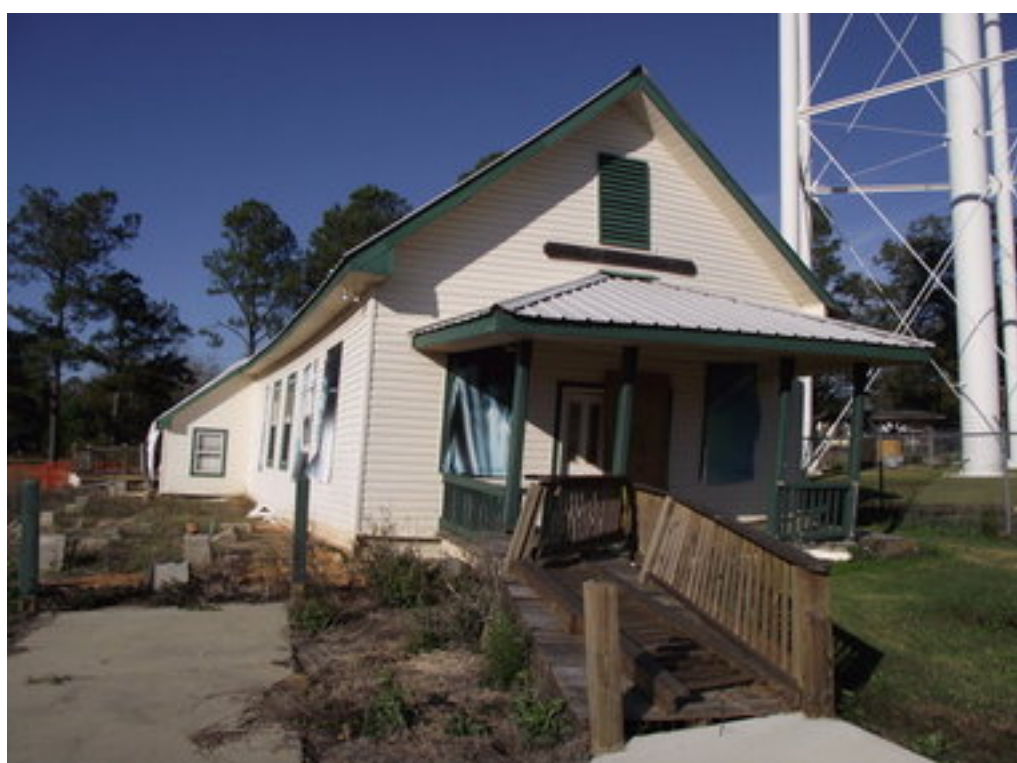
The Little Hall in Silverhill was damaged by a tornado in March. Residents are working to restore and move the 91-year-old building. (Guy Busby/Press-Register)
